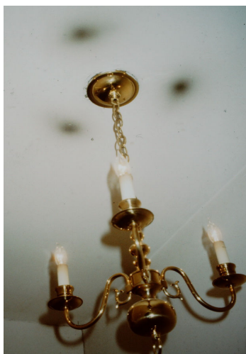
Soot stains on ceiling above light May Indoor Air Investigations LLC
